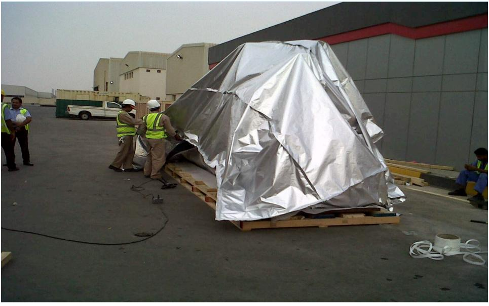
Air Filled to check leakage
